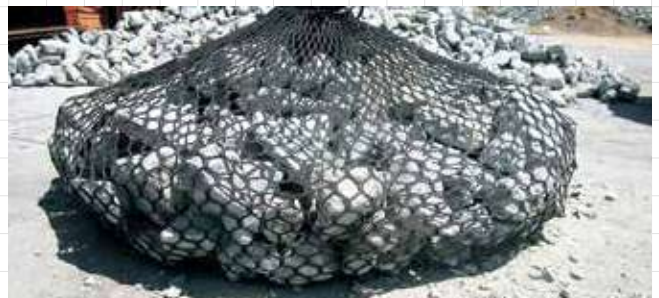
6 Placing at temporary storage
