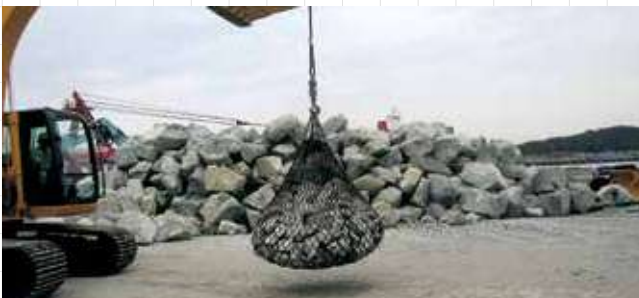
5 Lifting and moving to temporary storage
